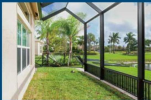
Construction Screen Installation
